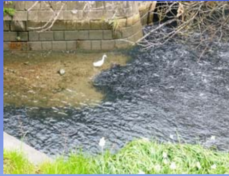
Photo by MK Architect Office Cheering Group
