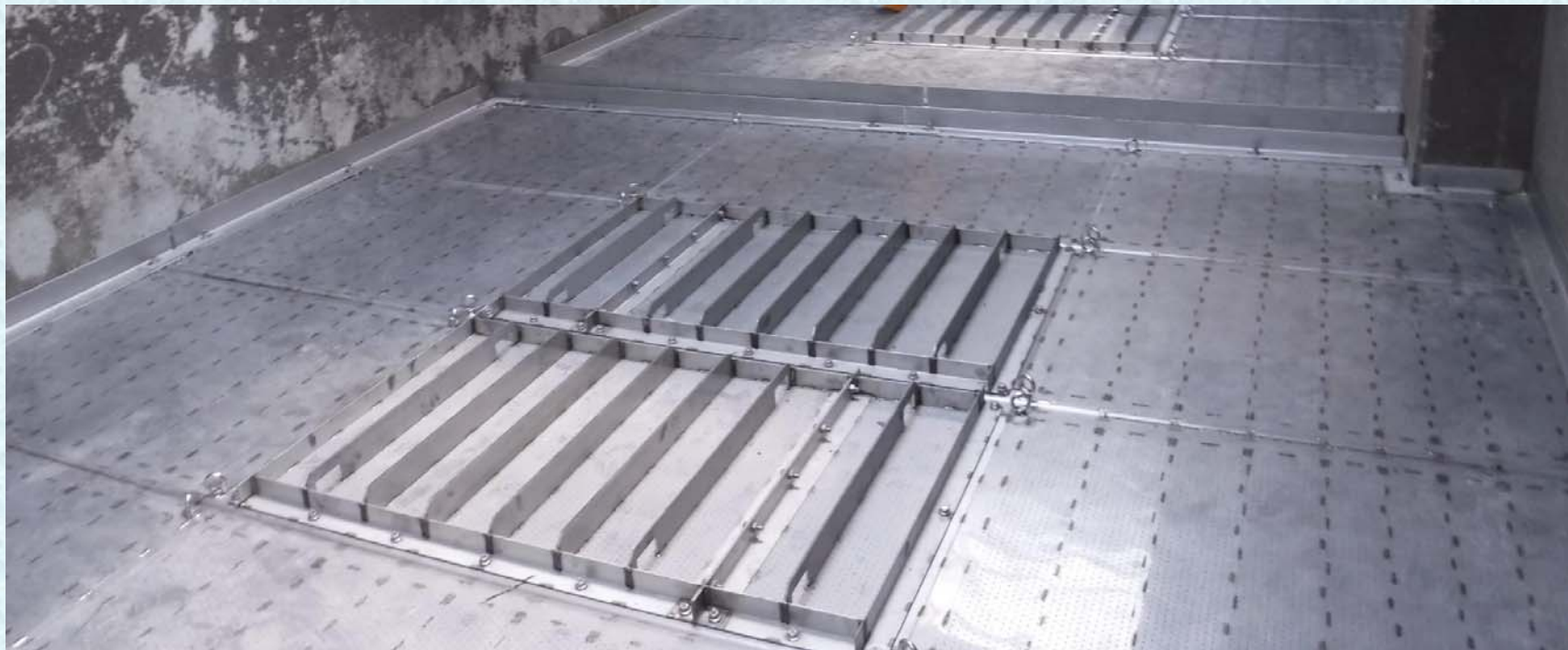
After facility renovation
