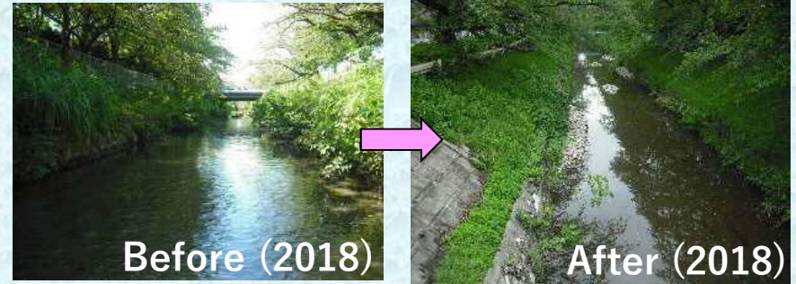
Construction in 2018 (Downstream of Kizune Bridge)
