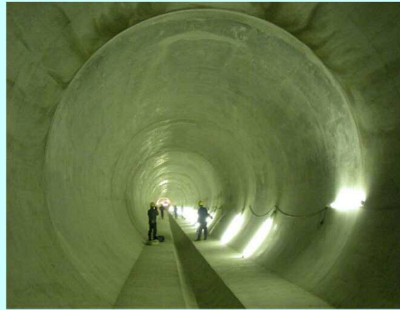
Horikawa -river right bank Rainwater Reservoir for pollution control
