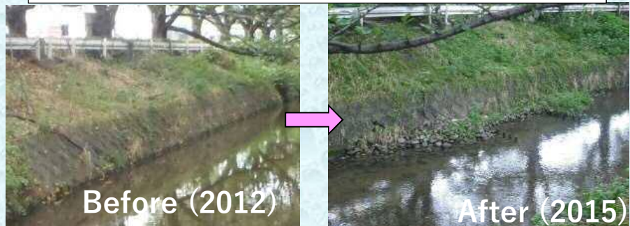
Construction in 2013 (Upstream of Kurokawa No.2 Bridge)
