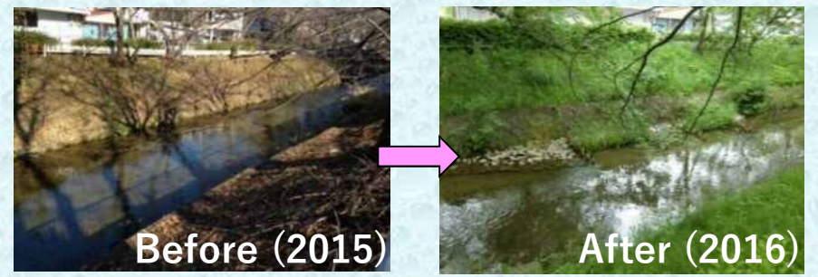
Construction in 2015 (Downstream of Ruriko Bridge)
