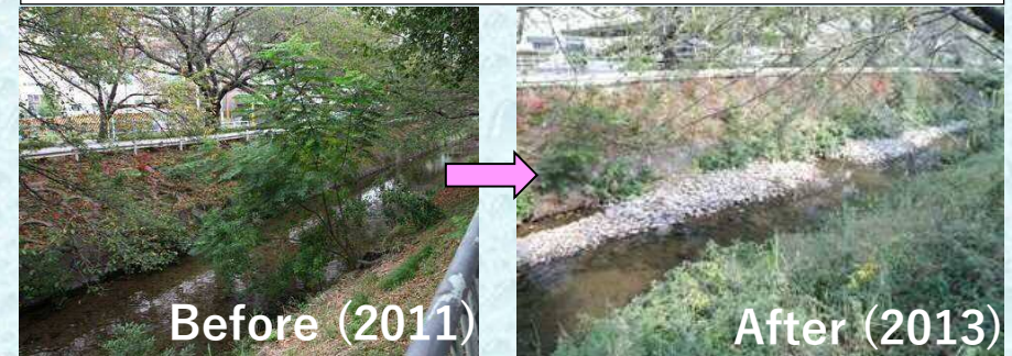
Construction in 2012 (Downstream of Kurokawa No.2 Bridge)
