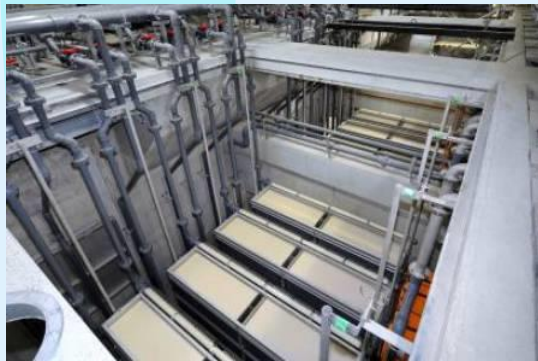
Flat membrane units in aerobic tanks (400 sheets × 12 units)
