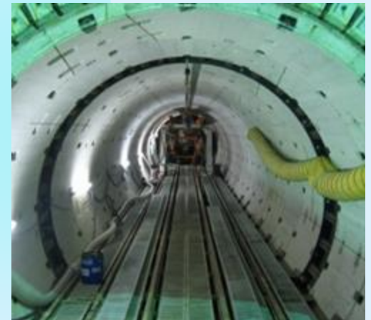
Under construction (14,000m 3 )
